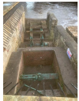
Cleared weir pit
